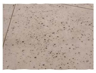
Figure 57: Potential Activity Node Pavement: Coloured Concrete Pavement with Salt Finish
