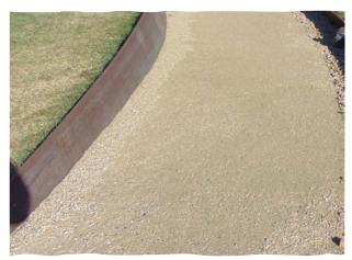
**Figure 56:** *Shared Path Pavement: Granitic Gravel with Cement Stabiliser*
