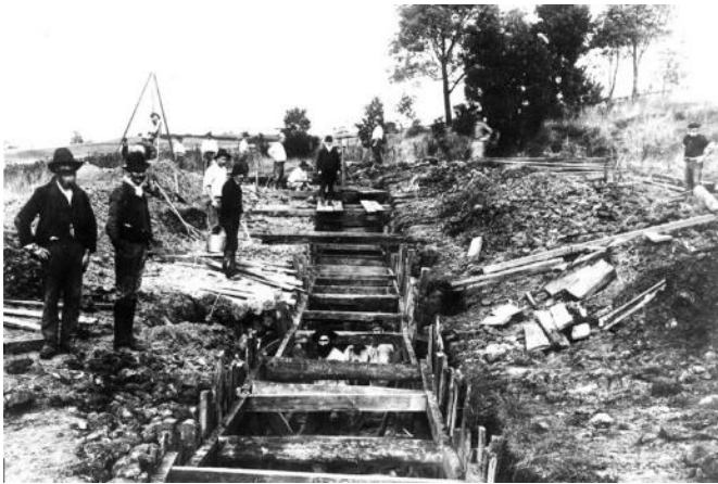
The construction of water races across hundreds of kilometres of Central Victoria took almost a decade. It was an extraordinary feat of engineering without the benefit of modern maps, GPS equipment or laser levels. Source: Coliban Water.
