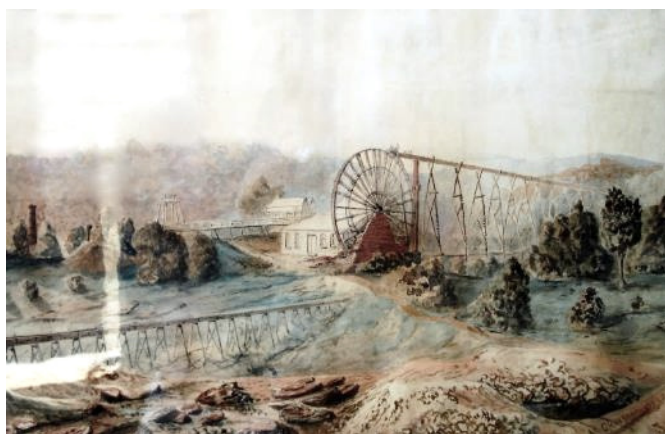
A watercolour painting of the Garfield Mine and Water Wheel from 1890 showing the headframe (poppet head) over the shaft (in the background, centre left) and the crushing battery and water wheel (centre) linked by the tram line. Two flumes can be seen: the one on the right carried water from the Coliban Water Race to the Garfield Water Wheel, and the one on the left carried the same water to the water wheel at Manchester Reef. The building behind the tramline may have been the Ebbott's house or the pump and winding mechanism for the shaft. Painting by Chas Marques. Source: Castlemaine Pioneers and Old Residents Association.
