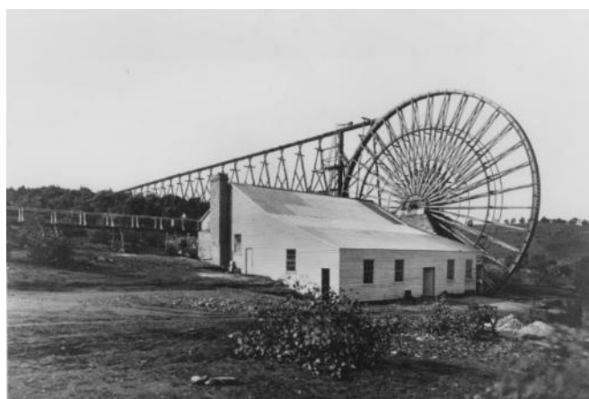
The Garfield Company water wheel and crushing battery. To the left of the battery is a raised tram line used to transport the heavy blocks of quartz from the mine shaft to the battery. Source: State Library of Victoria
