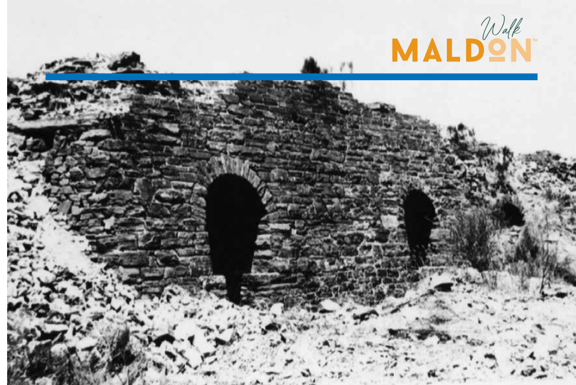
These quartz roasting kilns were located at Union Hill Mine, but were demolished in 1990-1991.
